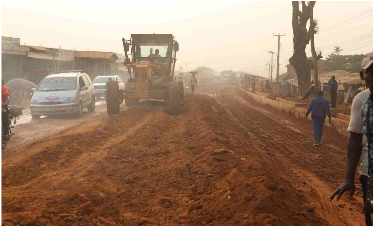
On-going Works at Lapai Axis of the Bida – Lambata Road
