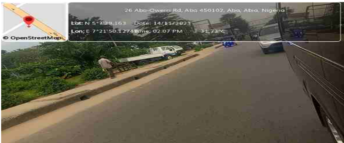
Fig. 11 Rehabilitation Of Aba-owerri Road
