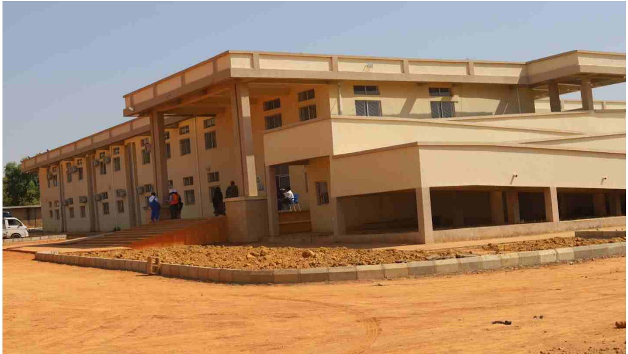
Front view of the Completed Construction of Amenity ward at JUTH
