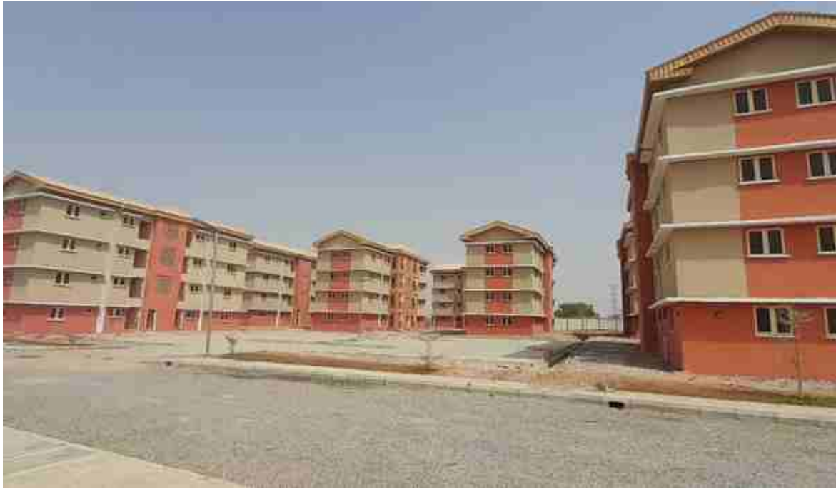
External view of the 5 numbers of 2-bedroom block of flats (blocks B6 & B7), Yola Command, Adamawa
