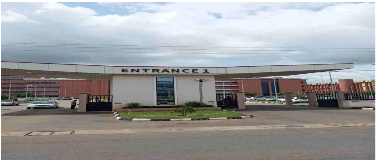
Fig. 10 Construction Of A New Central Secretariat Asaba.
