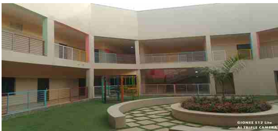
Completed Paediatrics Complex at ABUTH
