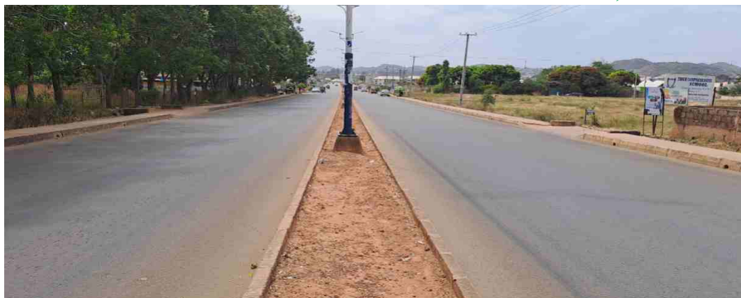
Fig. 8 Old Airport Road Junction, Ray Field, Bukuru Road
