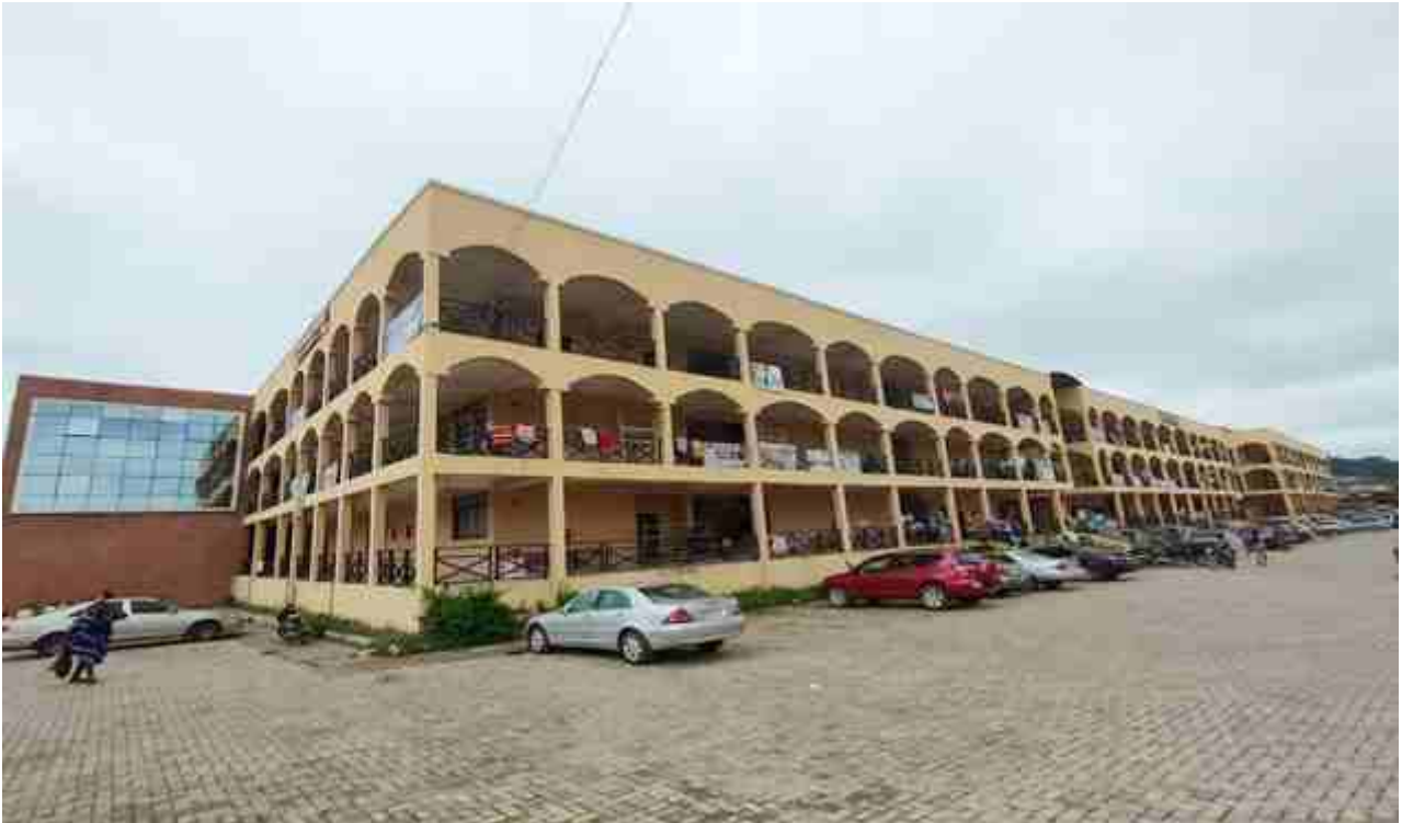
Fig. 12 Completion Of The Ultra-modern Oja Oba Market, Ado Ekiti.
