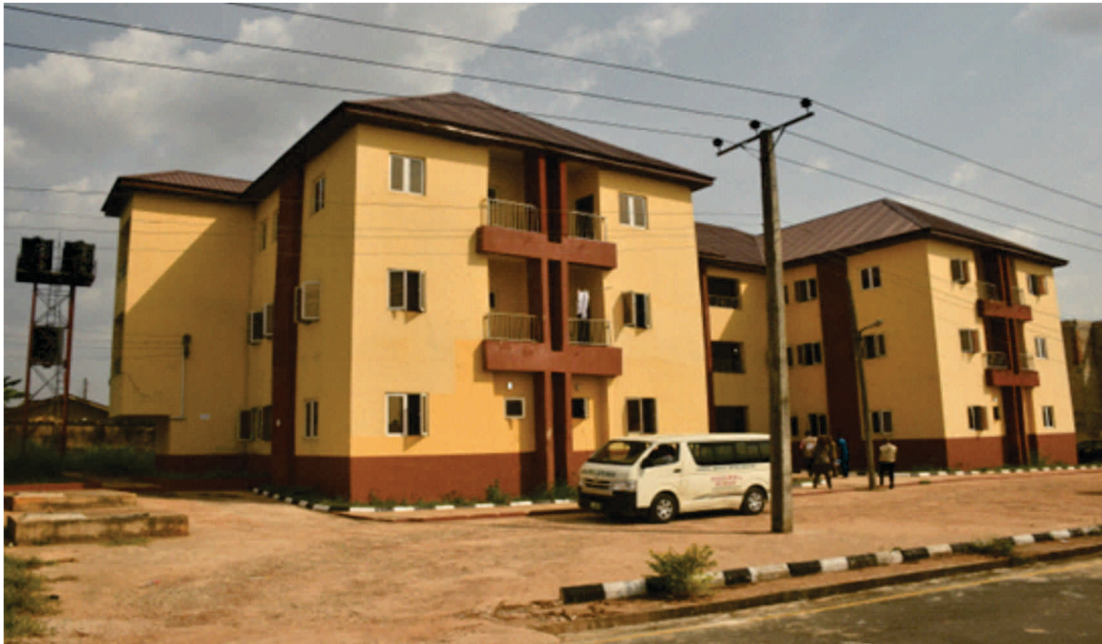
Fig. 47 Completed two storey house officers building with flats FMC, Umuahia, Abia state
