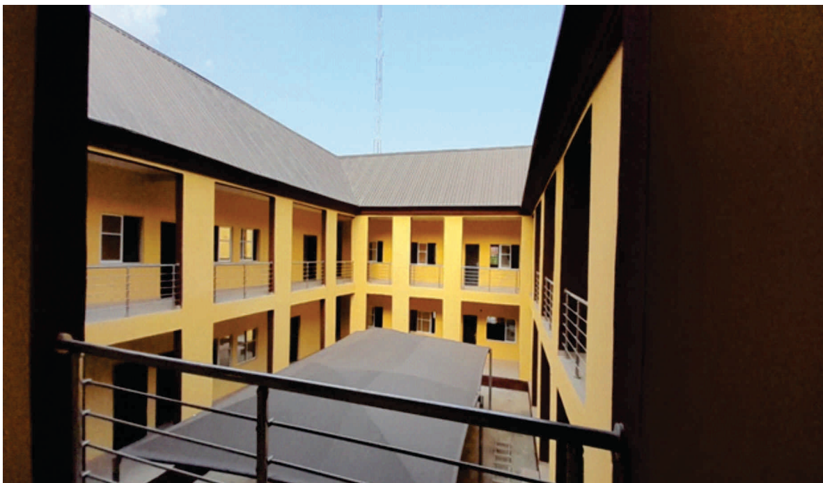
Fig. 65 Overview of the completed NIS Command Office Complex, Akure, Ondo state
