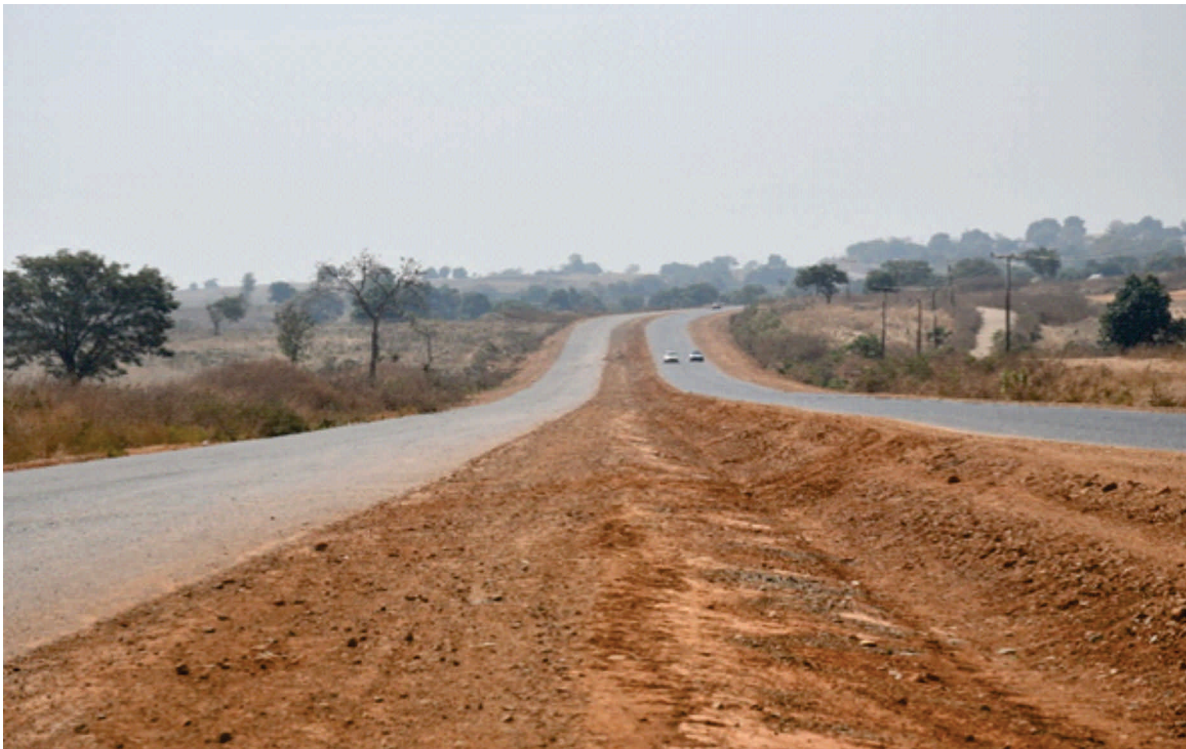
Fig. 1 Stretch of the constructed carriageway of the Suleja-Minna road in Niger State
