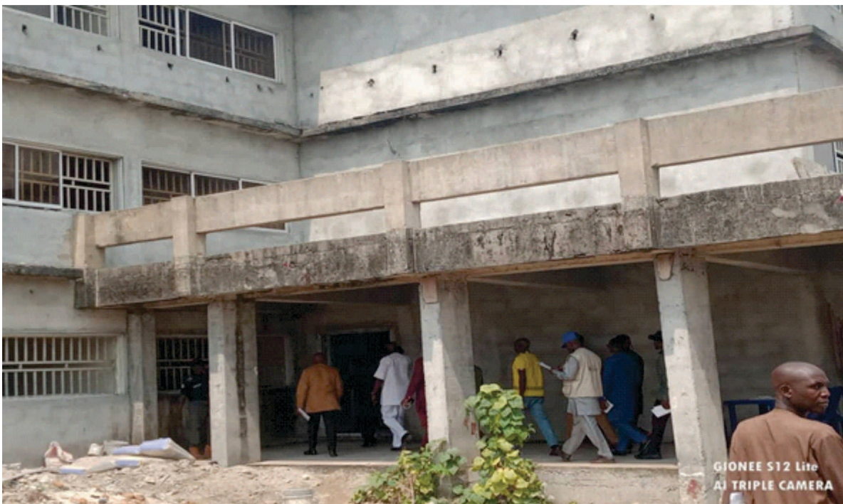
Fig. 55 Entrance to the ENT Building UPTH, Rivers State
