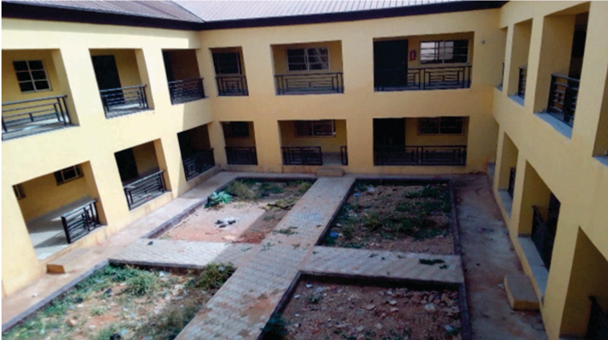
Fig. 20 Inner view of the Command Office Complex, Gombe State
