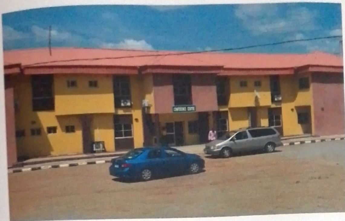
Frontage of the Trainee Hostel Block/Conference Centre, NCAM - Ilorin
