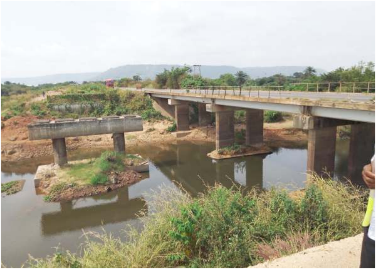
One of the Completed Bridges at Section IV Koton Karfe-Logoja Road
