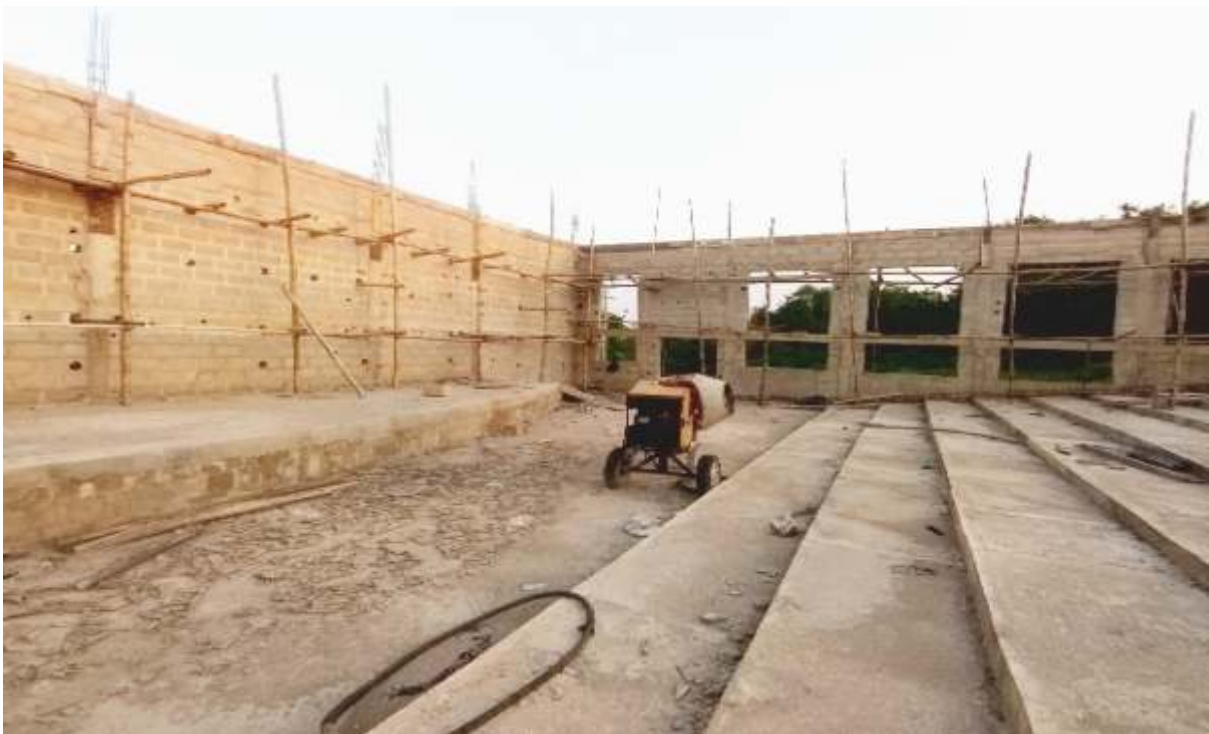
On-going Construction of 1000 Capacity Lecture Theatre at FCA, Ibadan, Oyo State
