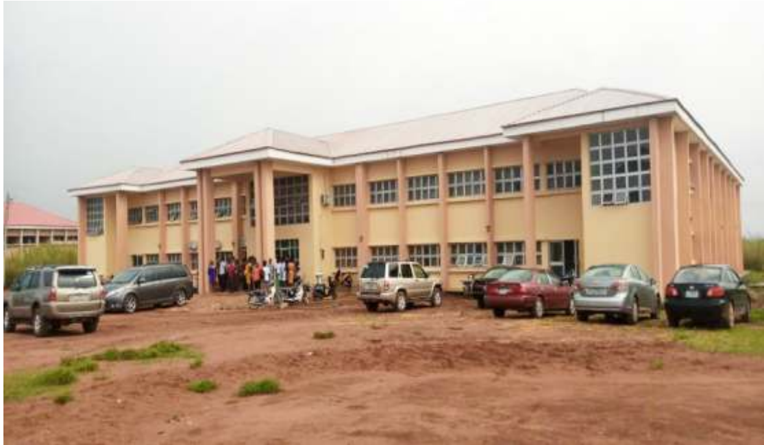
A Cross-Section of the completed Specialty Clinic at the Nnamdi Azikiwe University Teaching Hospital, Nnewi, Anambra State
