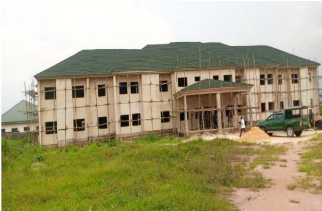
Ongoing construction of SHQ office of NCS at Umuahia, Abia State
