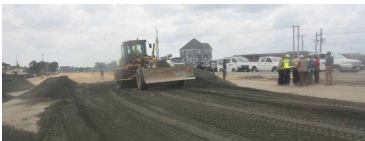
Soil-cement Sub base compartment on-going on the Enugu-Umuahia-Aba-Port Harcourt Express-way
