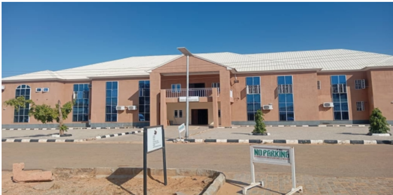
Fig.19 Completed construction and equipping of the Eye Specialty Complex at the FMC, Birnin Kebbi, Kebbi State
