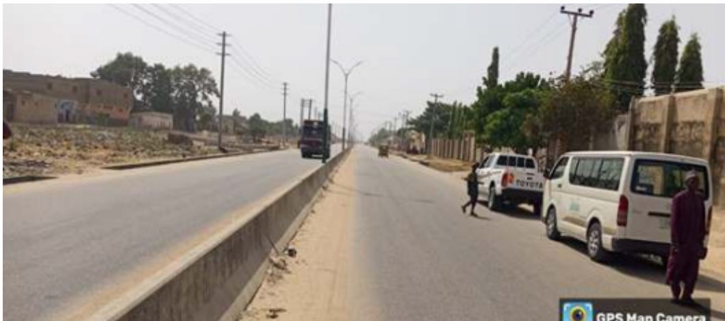
Fig 32 : Completed dual carriage access road with street lights to Dala Inland Dry Port, Zawachiki, Kano, Kano State
