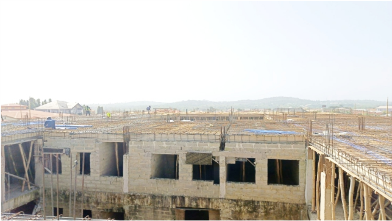
Fig.22 On-going construction of 150 bedded wards at Federal Teaching Hospital, Ido-Ekiti, Ekiti State
