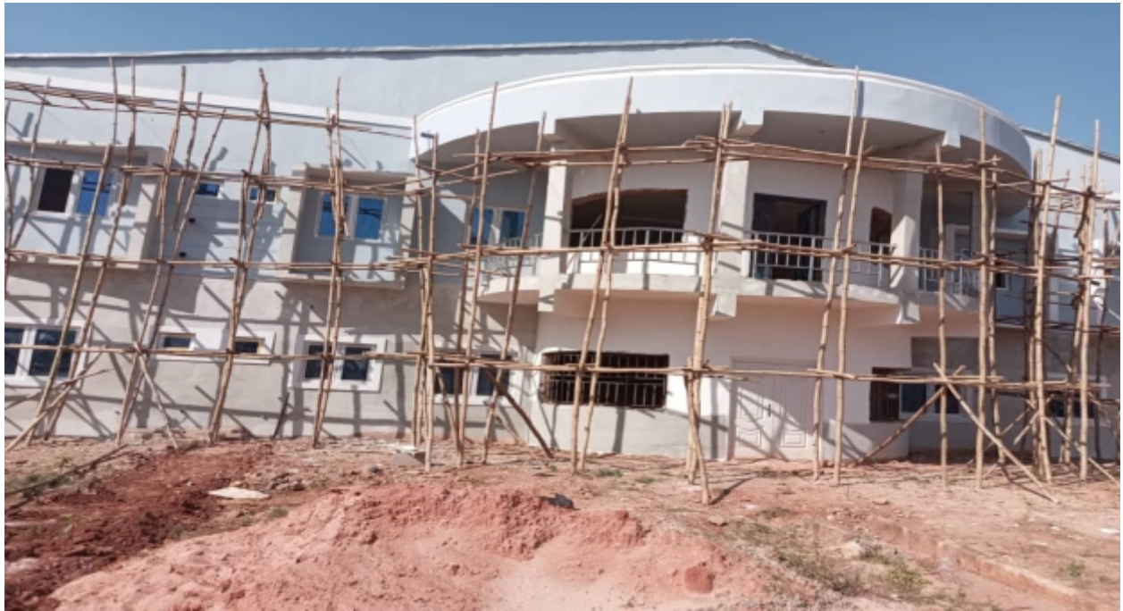
Fig. 21 Children's Emergency Isolation ward at Irrua Specialist Teaching Hospital, Edo State
