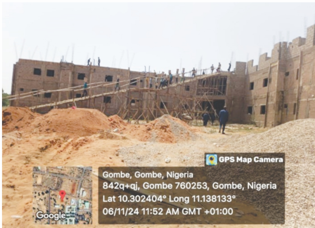
Fig.18 Laboratory Complex, FTH Gombe, under construction at FTH Gombe
