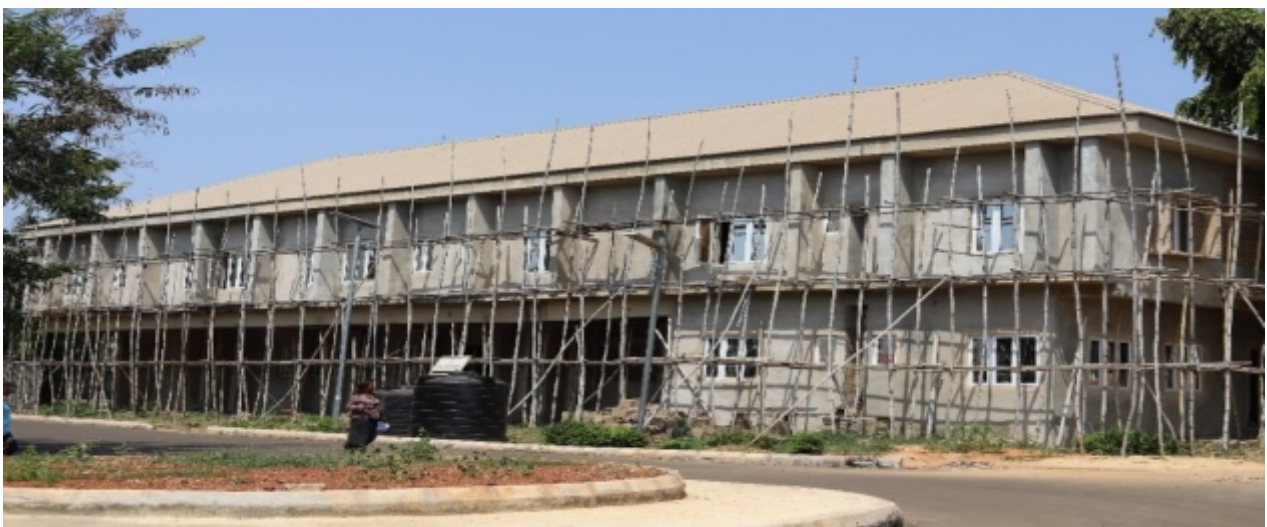
Fig.20 On-going construction of Students Nurses Hostel at Federal Neuropsychiatric Hospital Enugu
